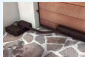
Above-ground motor, positioned to the side (when space is an issue).
