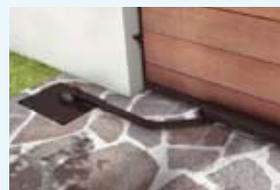
Below-ground motor in standard position.
